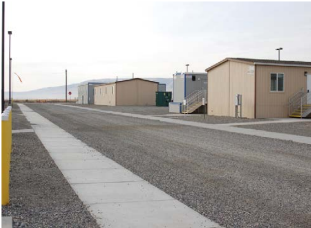
Figure 2: Mobile office areas include permanent sidewalks, lighting, roadways and utilities.
