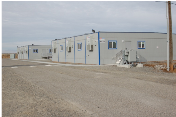
Figure 1: Five-wide modular offices.
