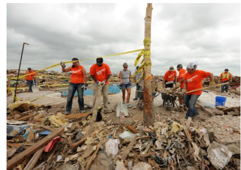
Debris Removal Operations after the Oklahoma Tornado. (Source: FEMA)
