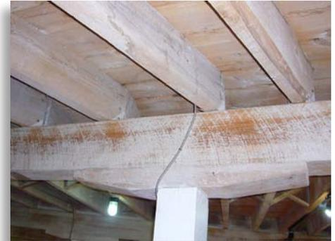
The thick wooden columns, beams, girders and floor deck are common elements of heavy timber construction (Type IV) that is noted for its slow burn times.
