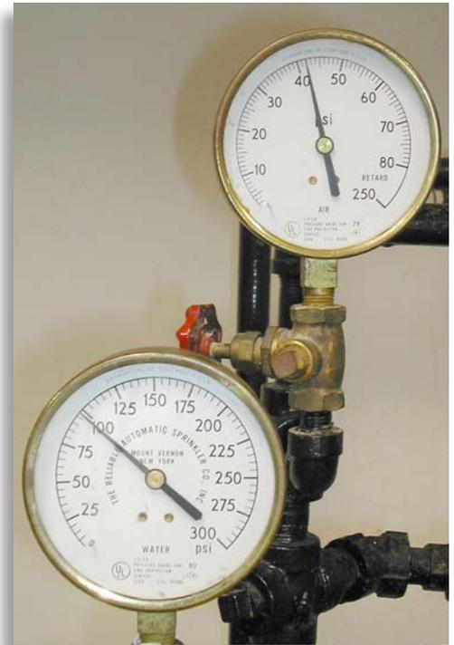
On this dry pipe system, the lower gauge measures the water supply pressure, and the upper gauge measures the air pressure maintained on the sprinkler system.
