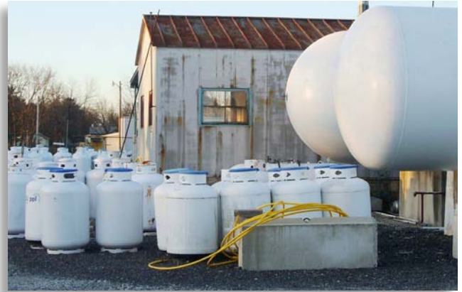
Separate structures used for indoor parking and servicing of LP-Gas transport vehicles by owner/operators must meet certain construction criteria.
