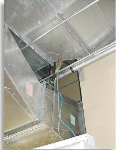
The cumulative width of these air handling ducts exceeds 4 feet (1.2 m), so the fire protection contractor has installed a sprinkler beneath them.
