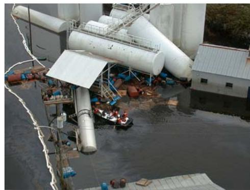
This bulk storage facility was damaged by floodwaters, potentially releasing dangerous flammable liquids. Photo courtesy of Federal Emergency Management Agency (FEMA)/Liz Roll.
