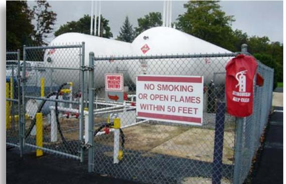
This fenced enclosure provides an additional perimeter of safety and security for this LP-Gas transfer system. Photo courtesy of McLaughlin's, Waynesboro, Pennsylvania.
