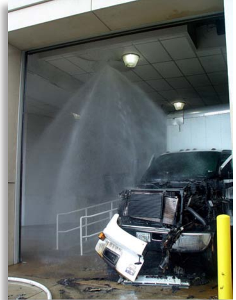
This control mode sprinkler is discharging a desirable pattern to control a fire by wetting nearby combustible materials.
