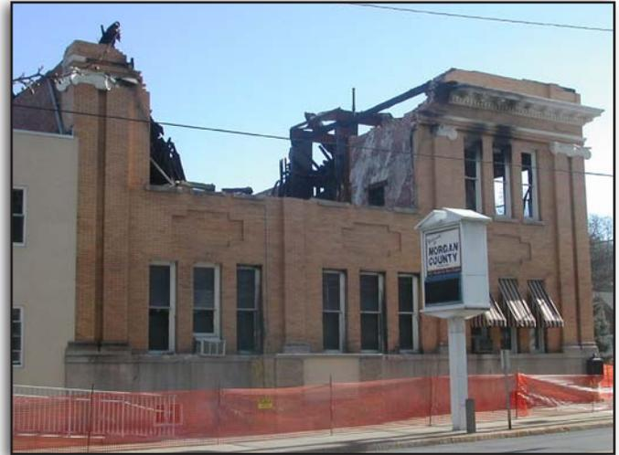
This burned out bank building shows an example of collapse in Type III construction.
