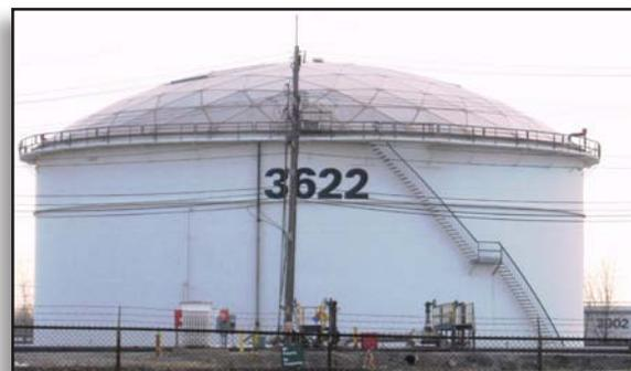
This bulk petroleum tank geodesic dome roof is made from noncombustible aluminum.
