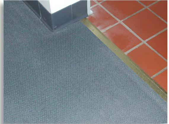
Depending upon the local codes, the combustible carpet in this picture may have to comply with Class I or II interior floor finish requirements.
