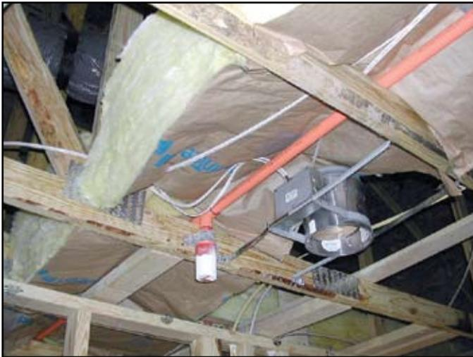
In this illustration, it also is interesting to note that the light fixture appears to be in direct contact with the Kraft paper backing. One might consider this as a potential fire hazard due to the heat emitted from the lamp. This particular fixture, though, is a Type IC rated fixture, and is Underwriters Laboratories (UL) listed for use in direct contact with thermal insulation.
