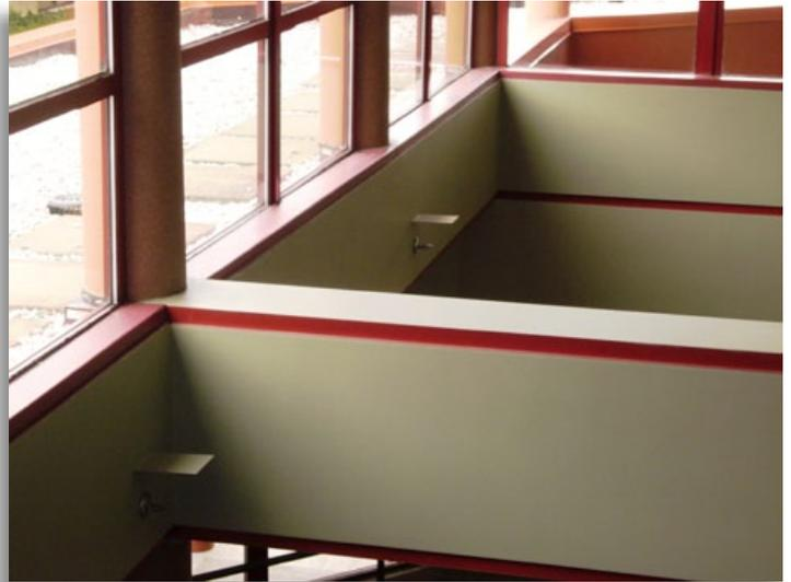
The small projections are intended to collect rising heat to operate the sprinklers in a timely fashion.
