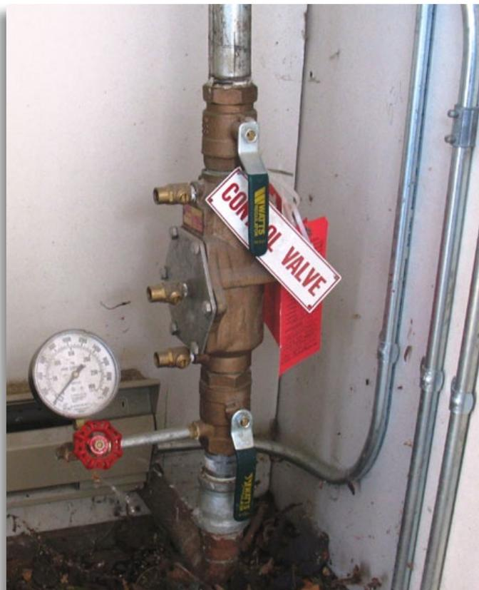
Photo courtesy Freedom Fire Protection, LLC, Longmont, Colorado. This residential sprinkler system has no water pressure, or the gauge valve is closed.
