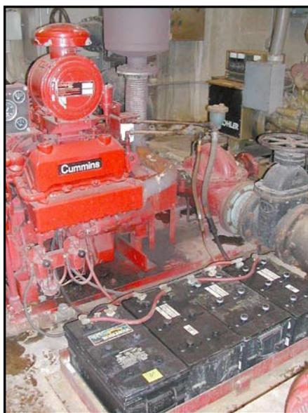
The storage batteries also must be equipped with two recharging power sources. One must be the generator or alternator furnished with the engine, and the other must be an automatically controlled charger that takes power from an alternating current power source such as a standard wall outlet. If an alternating current power source is not available or is not reliable, another charging method must be provided as the second source.
