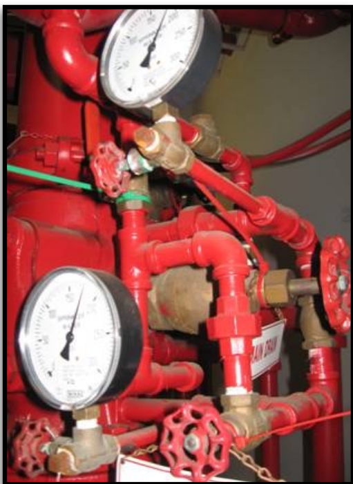
These simple plastic ties mark the valves' “normal” position. Photo courtesy James M. Robinson, University of Maryland.
