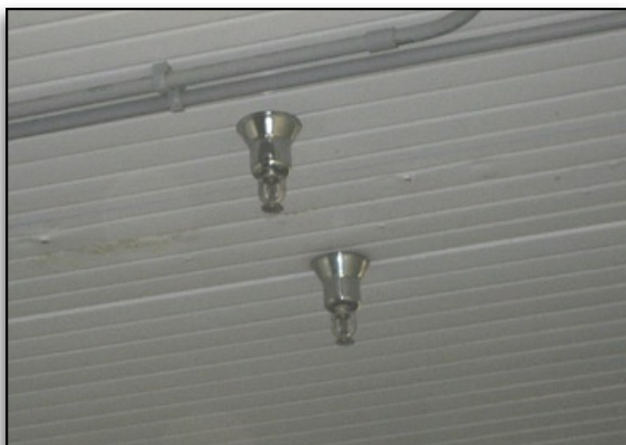
These sprinklers should have a baffle between them. Photo courtesy Minnesota State Fire Marshal's Office.
