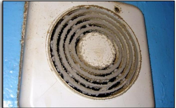
The dust accumulation on the face of this fan cover suggests that the electric motor behind it may be dirty as well.
