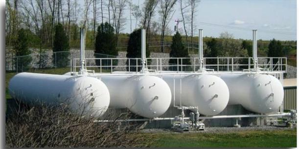
Photo courtesy Eastern Propane & Oil, Hudson, New Hampshire. In some instances, as many as nine of these bulk LPG containers may be arranged together.
