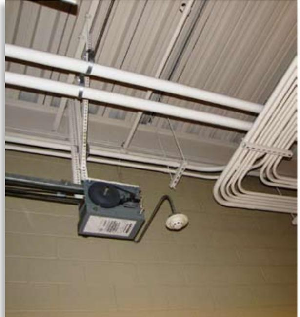
The placement of this spot-type detector should be evaluated by the code official to assess its potential performance.
