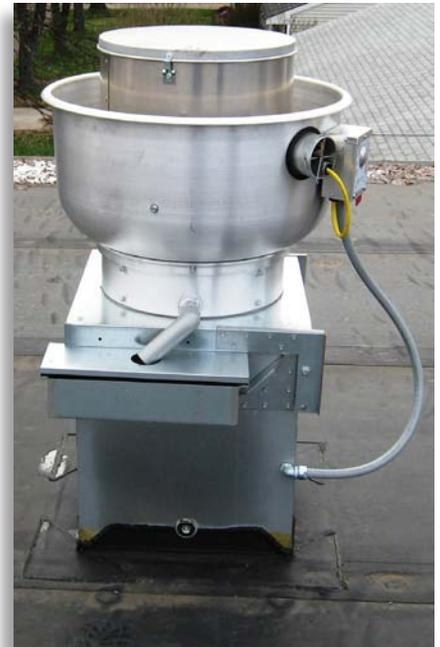
This newly installed rooftop exhaust is an example of an upblast fan assembly from commercial cooking equipment where grease-laden vapors are created.
