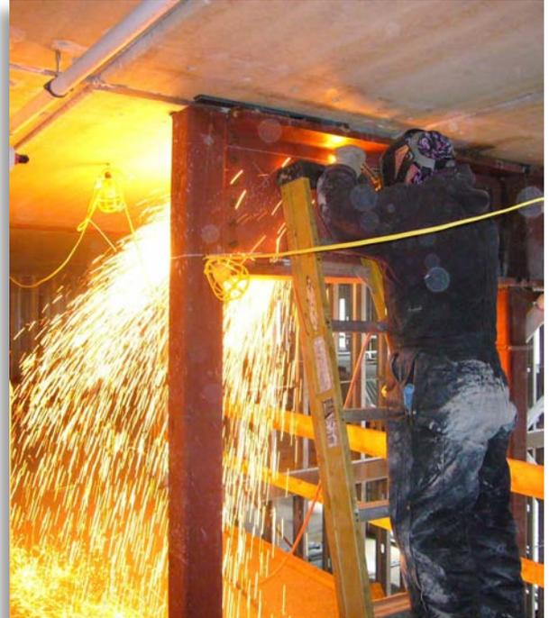
Sparks and slag from hot work operations are a common source of unwanted fires.
