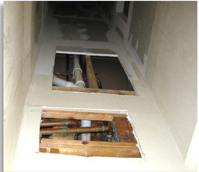
The openings in this fire-resistive-rated shaft should be repaired to control fire spread. *Photo courtesy R. Wayne Powell, Marriott Corporation.*
