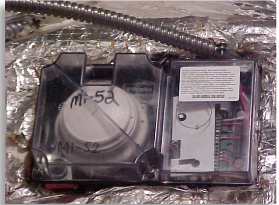
This smoke detector assembly is mounted on the outside of a duct system and employs sampling tubes in the air stream to collect smoke particulates and carry them to the detector's sensing mechanism.
