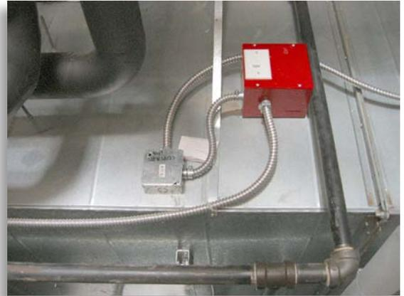
The exterior-mounted duct smoke detector is mounted on a large duct, so additional duct detectors may be required.
