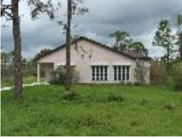
"Hurricane House" at Fort Pierce incurred no structural damage during Hurricanes Frances and Jeanne.
