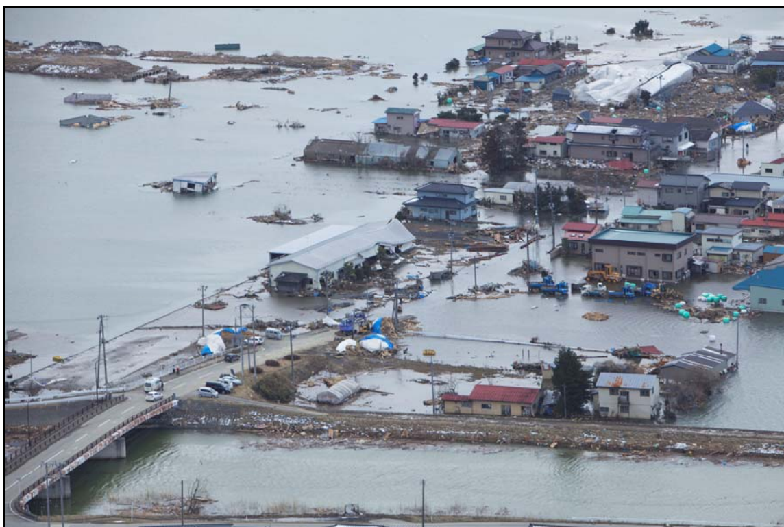
Figure 8. Aerial View of Minato, Japan, a Week After the Tsunami
