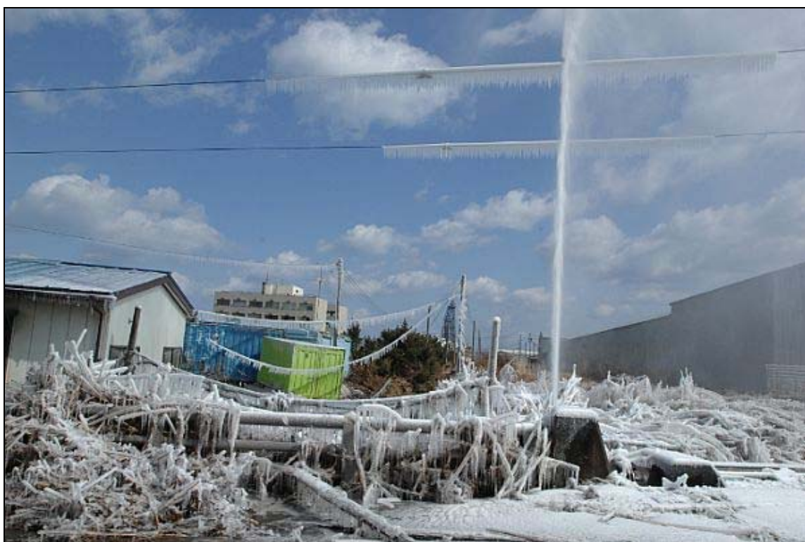
Figure 7.A Damaged Water Pipe Shoots into the Air, Hachinohe, Japan
