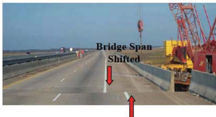
Figure 3: I-10 Bridge Repair at Pascagoula
