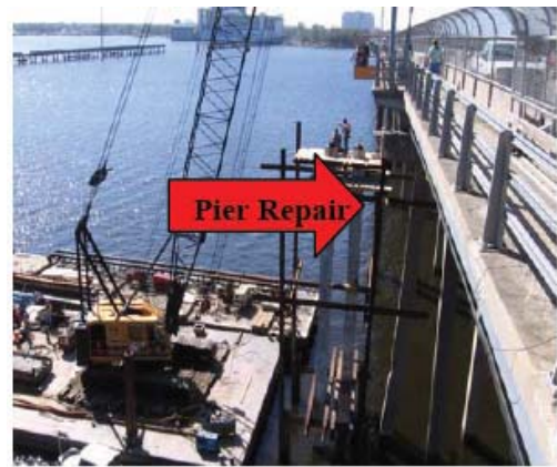
Figure 6. I-110 Bridge Repair
