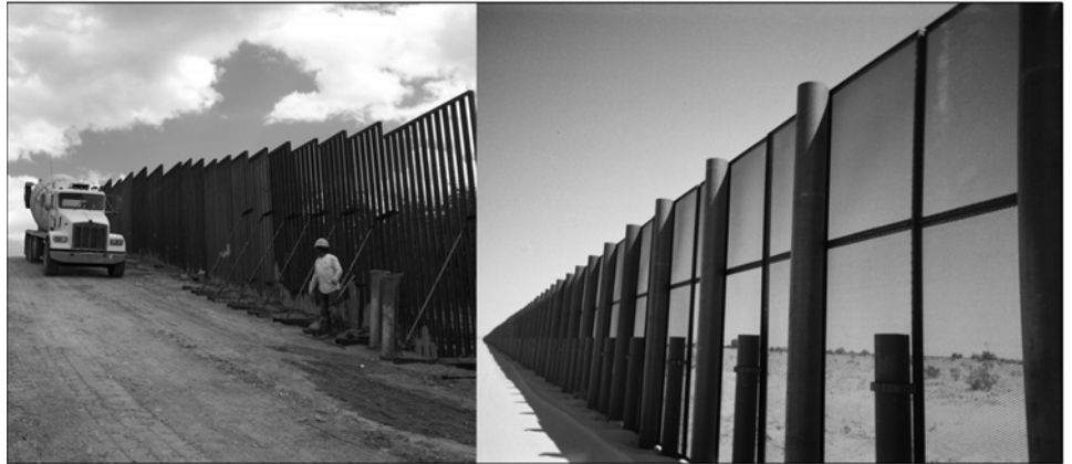
Figure 4: At Left, SBInet Fencing Being Deployed at Sasabe, Arizona; at Right, SBInet Fencing Deployed at Yuma, Arizona
