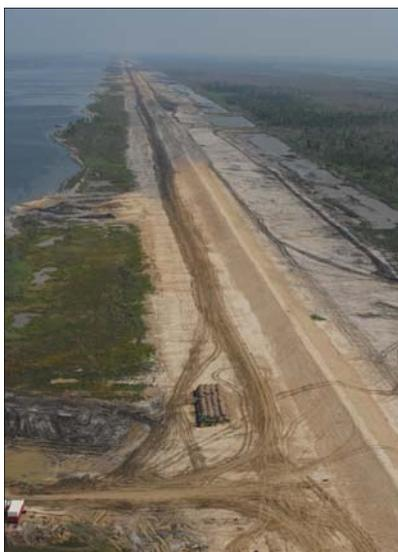
**Millions of cubic yards of soil will be needed to restore and build the levee system in the greater New Orleans area; and all soil used is stringently tested.** (USACE Photo)
