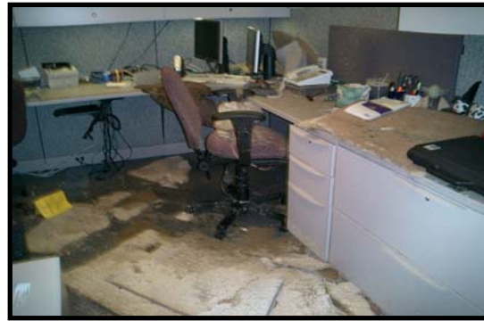
Damage inside MMS building Photo Courtesy of MMS
