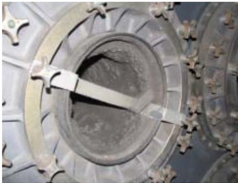
Figure 6. Cylindrical CBR Pre-Filter Retention Bar Incorrectly Installed Over a Bag Pre-Filter
