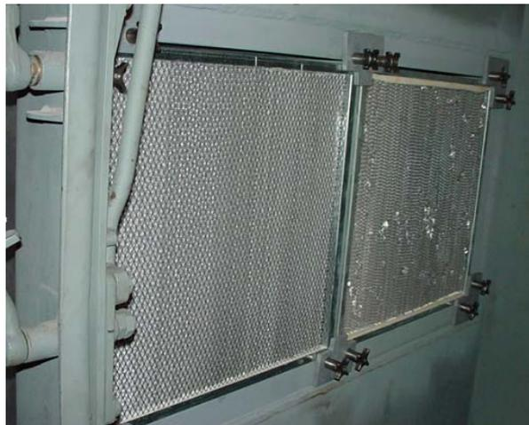
Figure 7. New LP HEPA Filter (Left Side) and Old LP HEPA Filter (Right Side)
