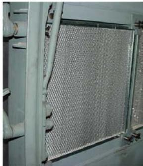
Figure 3. 2000 CFM LP HEPA Filter Installed
