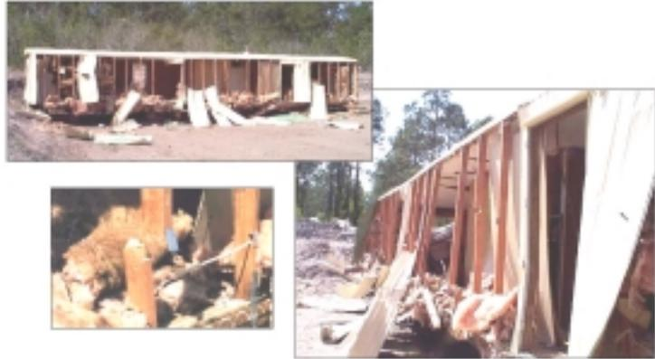
**Figure 3. Damage from 12 psi Bomb Blast**
