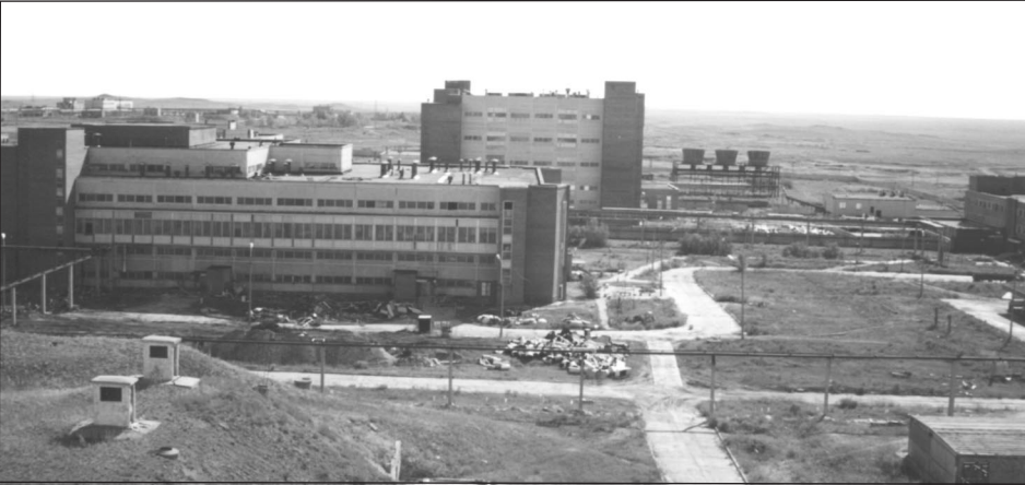
Building 600 (foreground) Research Facility and Building 231 Anthrax Milling and Drying Facility.
