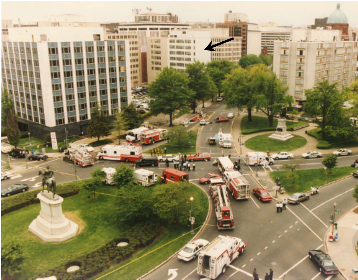
Photo 7. An overview of apparatus placement. The arrow points to the B'nai B'rith Building.
