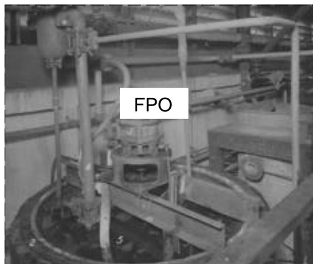
**Fig. 2-21.** Interior view of the Phosgene Production Plant at Edgewood Arsenal, Md. The low level of chemical engineering technology apparent in this World War II-era photograph is relevant to the problem of chemical agent proliferation today. Elaborate, expensive equipment is not required for mass-producing the less-sophisticated chemical agents. Photograph: Chemical and Biological Defense Command Historical Research and Response Team, Aberdeen Proving Ground, Md.
