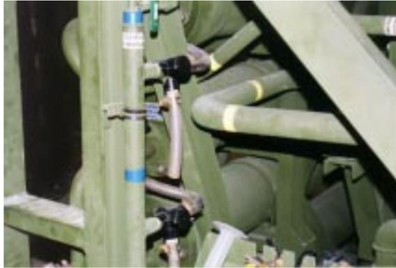
**Figure 37. Chemical Feed Run/Prime Values in PRIME Position.**
