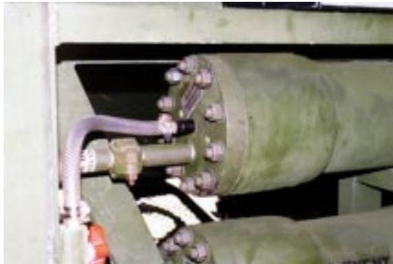
Push puller rod assembly through the center of the first end connector, R.O. element, interconnector, second R.O. element and out through the second end connector (figure 49). Secure puller plate on the end of the puller rod (figure 48). Double check to ensure you will be pulling elements out in the direction of product water flow.
