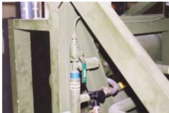
**Figure 35. Front R.O. Pressure Tube Vent/Sample Valves.**
