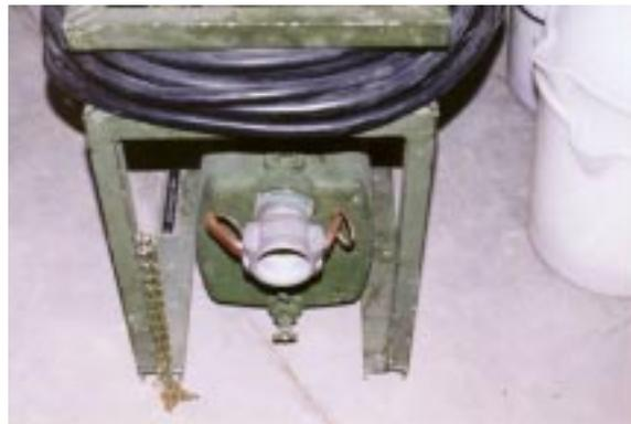
Install 1 ½-inch male quick disconnect fitting on discharge coupling of raw water pump #1 (figure 22). Ensure drain and vent valve on pump are closed.
