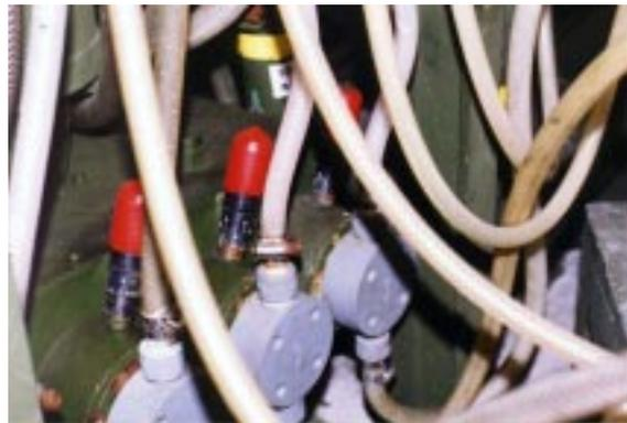
With the chemical feed pump operating, disconnect the return line from the POLYMER tank and flow the POLYMER into a 100ml cylinder for one minute. Measure the amount of POLYMER in the cylinder.
