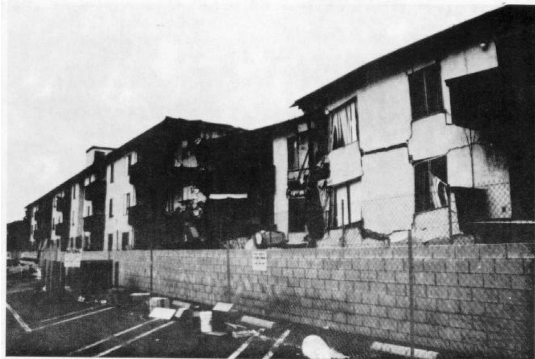
**Collapsed portion of Northridge Meadows Apartments. Due to the soft story construction, the structure not only collapsed, but shifted 10 feet.**
