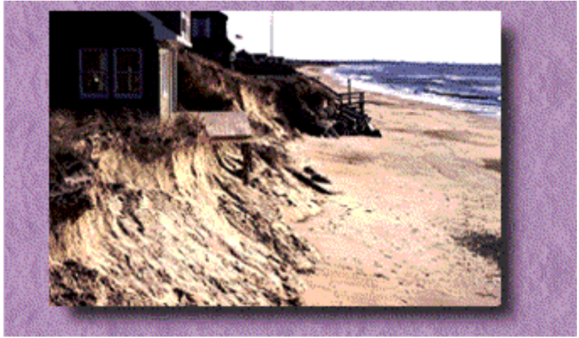
Photo 14. Folly Beach, South Carolina is plagued with erosion problems.
