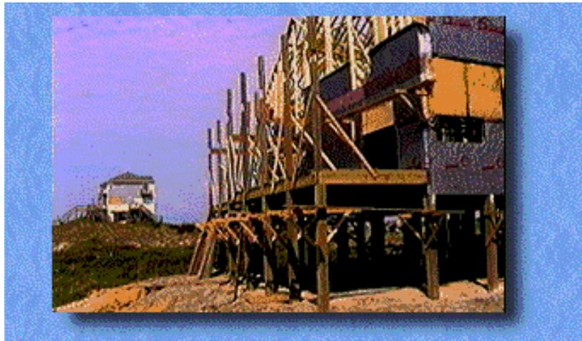
Photo 6. This house is being built on pilings to reduce potential damage from flooding and high waves.
