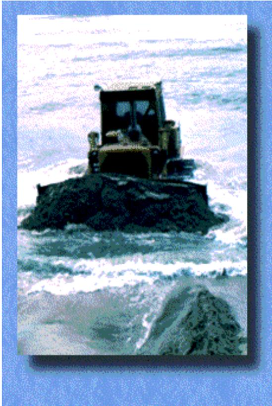
Photo 7. A bulldozer pushes sand onto the beach to rebuild the dune that helps protect the property behind it.
