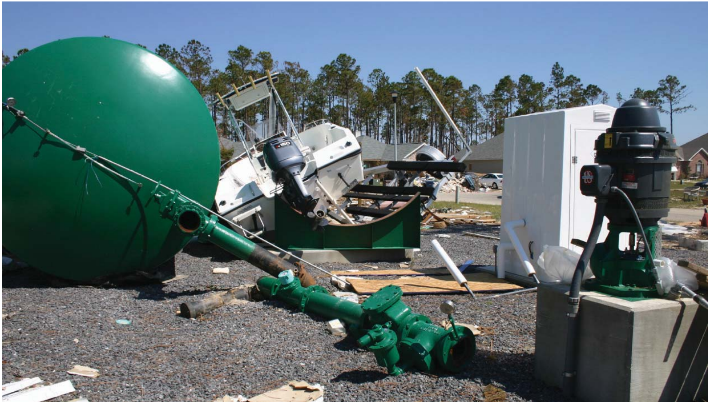
Destruction in the wake of Hurricane Katrina
