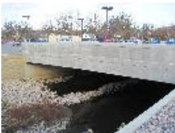
clear span bridge that replaced culverts that were too small to provide adequate water flow
