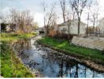
a portion of Pigeon Creek's rock-lined low flow channel and newly constructed retaining wall.
