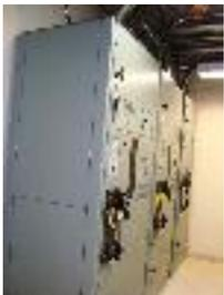
Photo of electrical utility units which were moved from the basement to the second floor of hospital
