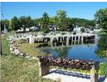
Perimeter weir overflow system type
