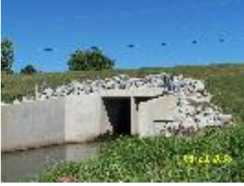
A dual box culvert
