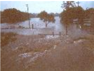
Water coming over dam
