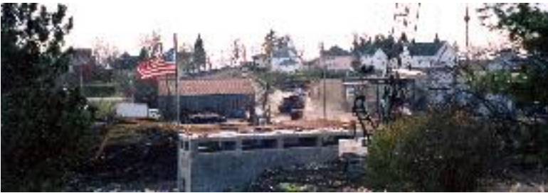
New dam in construction
