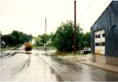
Tarrant Lake (to the right of the road) begins to overflow its dam during heavy, persistent rains in late May 1993.
