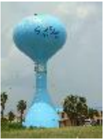
Dolly blasted paint off of South Padre's water tower
