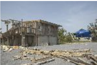
Dolly damaged many South Padre buildings, some severely
