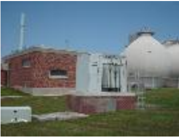
West transformer mitigated by raising the structure three feet
