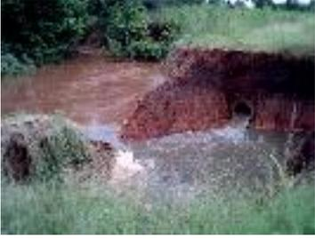
Duncan Sewer Failure - Creek wall breach
