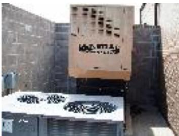
Masonry fence which protects the generator from flying debris
