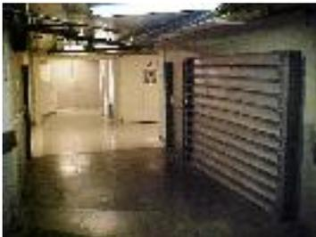
Picture of flood logs in front of door
